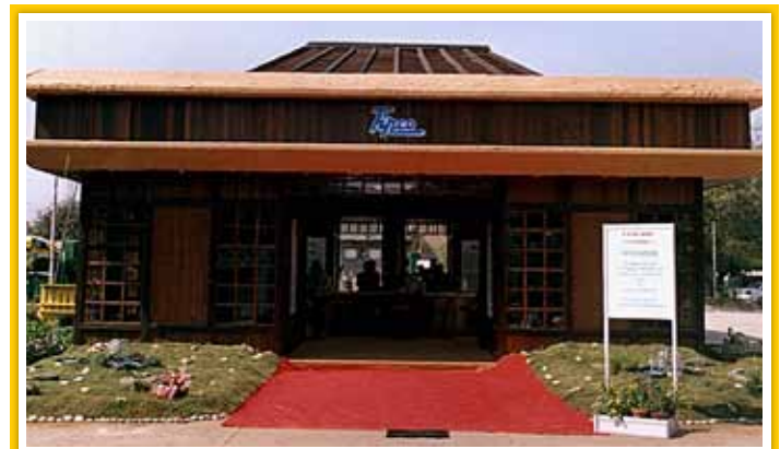
LARGE OUTDOOR STRUCTURES
