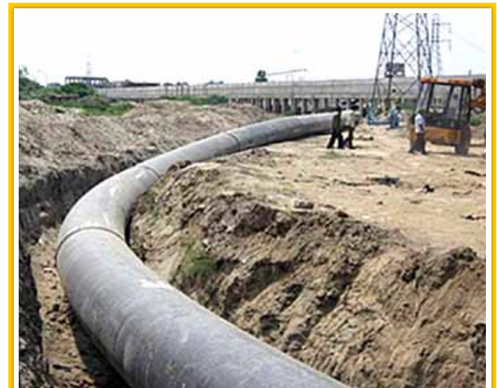
Fig. 12 1200 mm PE pipes for Sewerage Force/Pressure Mains in Delhi
