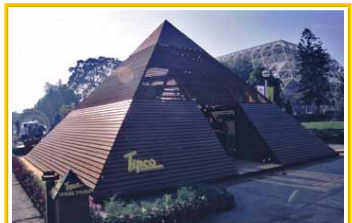
LARGE OUTDOOR STRUCTURES
